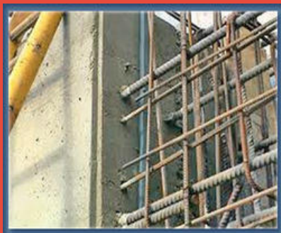
RCC Drilling
