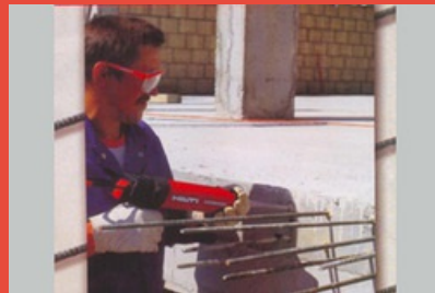
Rebar Fixing Service
