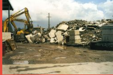
Rock Breaking Work
