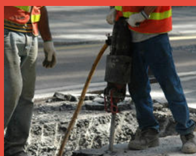
RCC Slab Cutting
