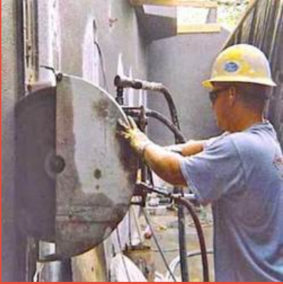
RCC Wall Cutting Service
