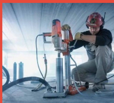
Core Drilling
